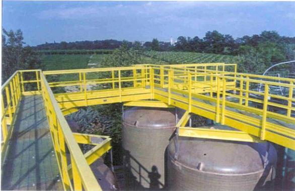
The FRP walkways are built by assembling fiberglass and polyester resin pultruded profiles and gratings; they assure several advantages compared to the normal metal ones:
